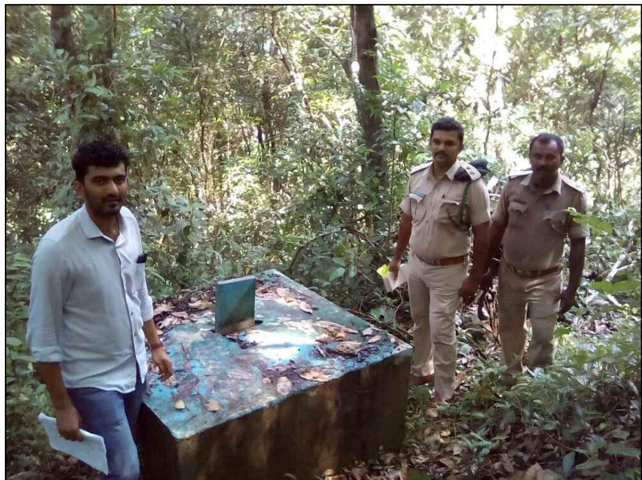
Photo 16: RCC structure for boundary marking, Puttur range, Mangalore division and circle
