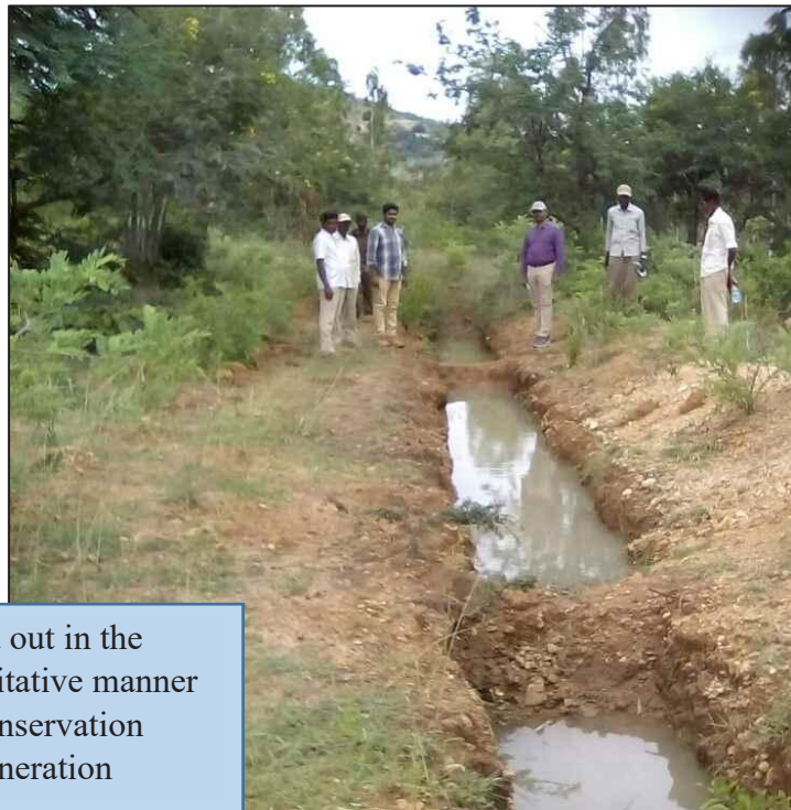
Photo 10: Surapalli plantation, Bagepalli range, Chikkaballapur division, Bengaluru circle Percolation trenches filled with water. Stabilised bunds with vegetation
